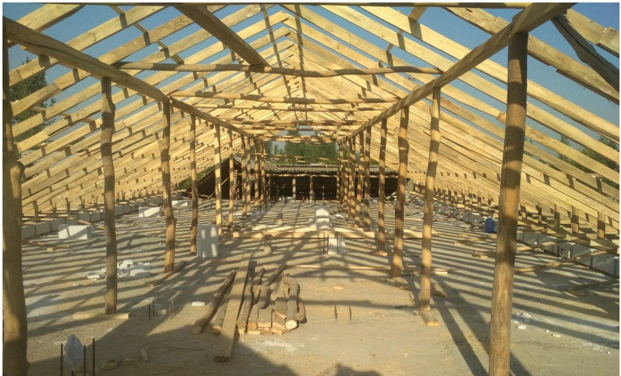
General view of wooden roofing elements .
