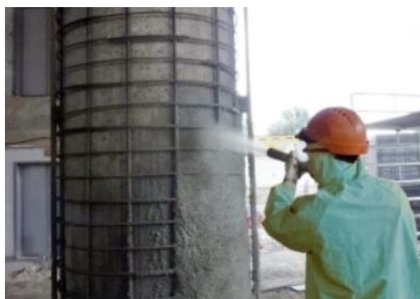
Figure 3. Technological process of strengthening a reinforced concrete column with a shell made of reinforced shotcrete.
