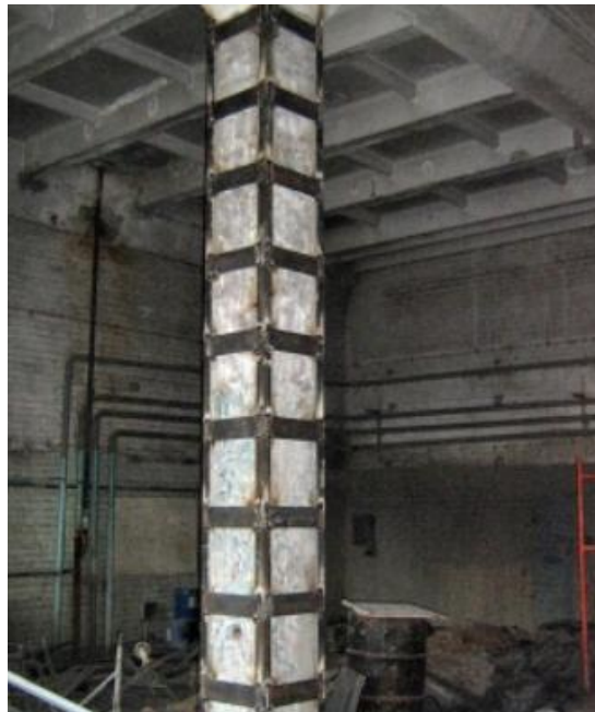
Figure 2. Strengthening a column using a steel shell.
